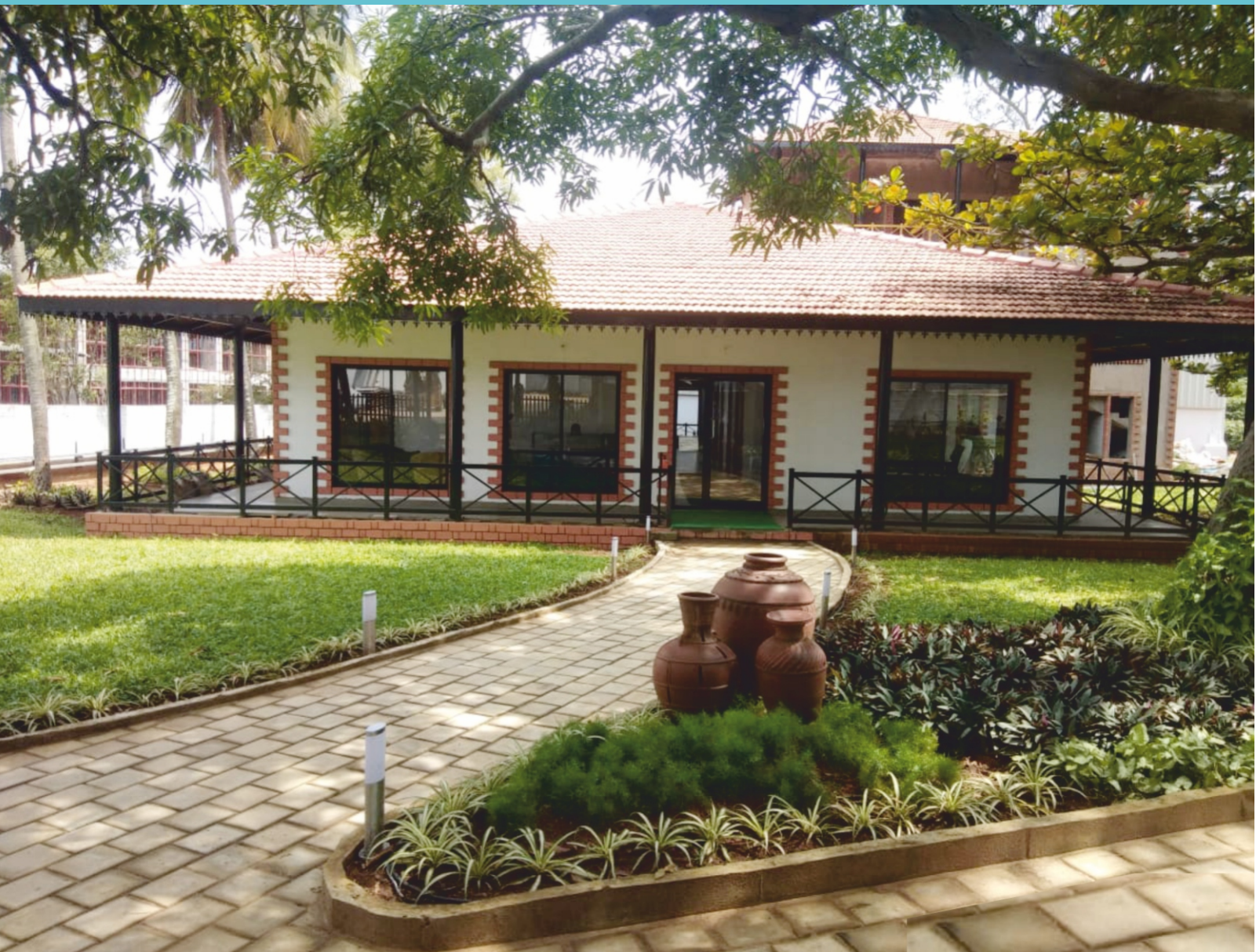
New Factory Administrative Office
